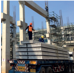
hollow core slab
